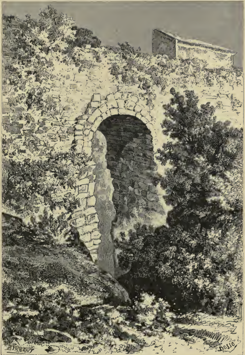
Bridge at Cora. 1
